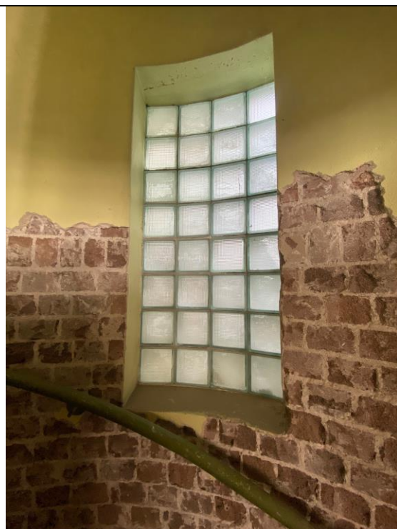
Figure 14. Glass brick window in stairwell, characteristic of geometric fashions in the interwar period. (Source: GML, September 2024)
