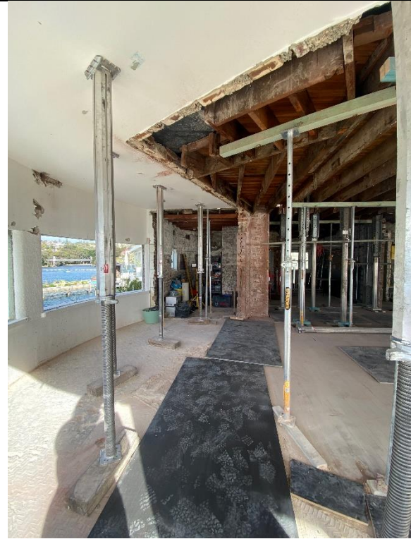
Figure 12: Ground floor looking southeast towards Parsley Bay. Extent of internal walls evident through the ceiling removal. Outline reflected in the ceiling indicate internal walls of earlier terrace shop, now removed. (Source: GML, September 2024)
